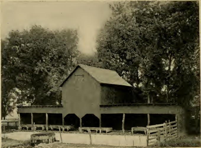
Fig. 14. Open shed and feed storage combined. In use by E. E. Chester, Champaign Co., Ill.
